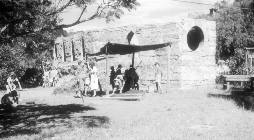
LEFT: ALFREDA HAZARD (WIFE OF THE HEADMASTER, IN GREY COAT AND SKIRT) CAN BE SEEN WITH THE MOTHER OF A PUPIL IN FRONT OF THE CHAPEL UNDER CONSTRUCTION.
