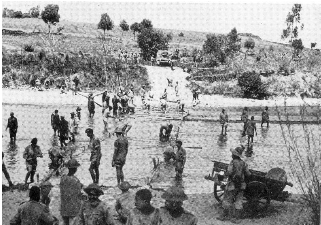
[LEFT: LAYING A BRIDGE ACROSS A RIVER NEAR ANDRIBA]
