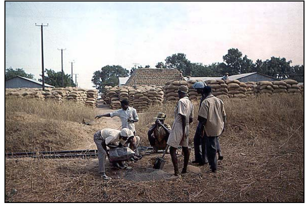
71. Finding 'safe' and useable locations for control beacons was not always very easy in busy areas. Here a beacon is being positioned on railway land near the groundnut stacking area at Gusau, Sokoto Province in 1961.
