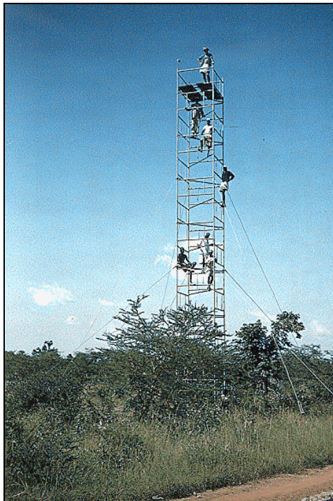
51. 'Home made' guyed towers constructed from Mills scaffolding were first used by Frank Waudby-Smith and Malcolm Anderson for the reconnaissance of a Tellurometer traverse from Kano to Nguru in 1961
