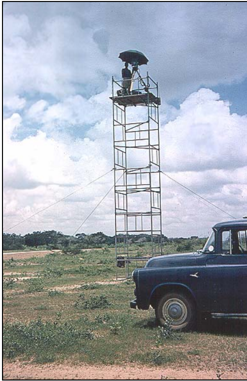
53. The modular form of the scaffolding allowed transportation of a moderately sized reconnaissance tower in a surveyor's 'kit-car'. Pictured at Jogana in Kano Province.
