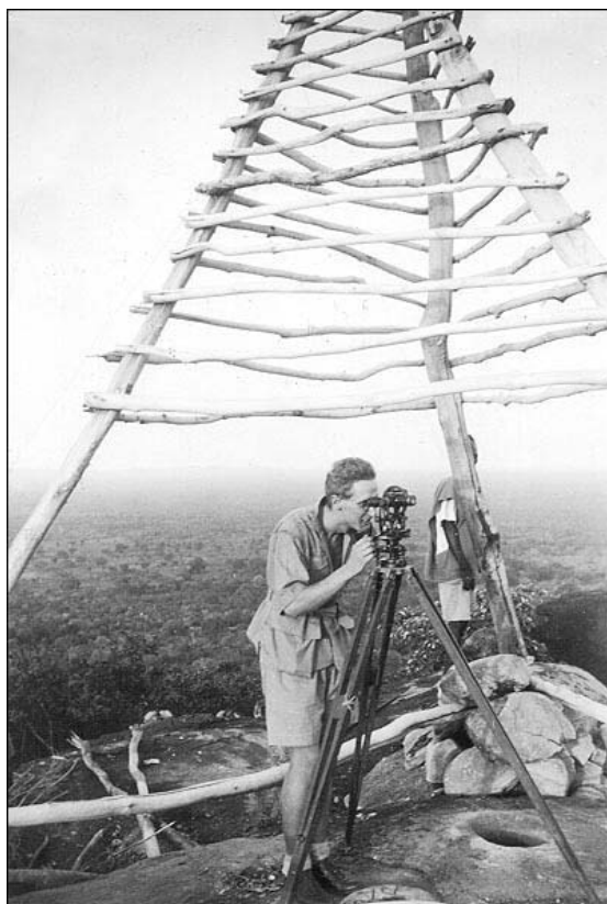
44. Keith Sargeant observing Tertiary triangulation in Katsina Province in 1939
