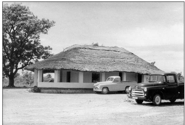
195. Wamba Rest House, with cement-plastered walls and floor and 'Crittall' window and doors frames with glass.
