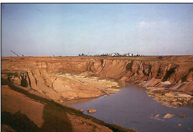
93. A deep mining pit at Rayfield; the aftermath of dragline working and used for water storage for sluicing operations.
