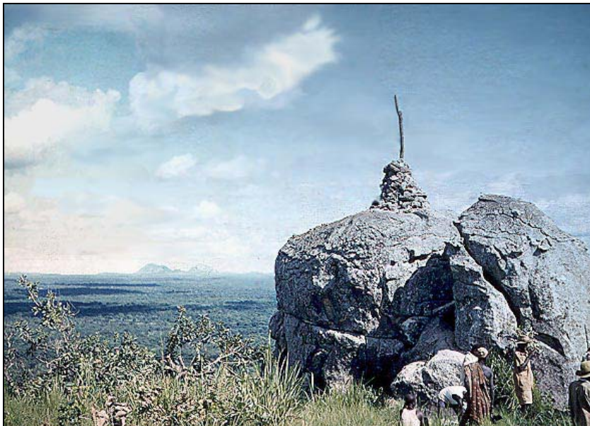
28. A site is chosen, and a temporary cairn erected, for a new point in the Jema'a secondary triangulation near Akwanga, Plateau Province, in 1957
