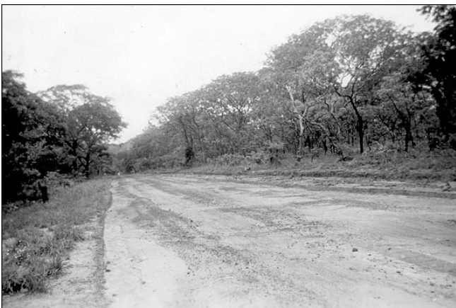
145. The main laterite-surfaced road from Kaduna to Ilorin in 1957.
